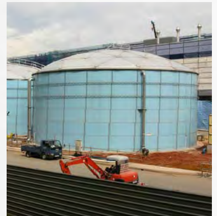
Industrial Service Water
