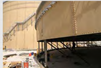
Jack and Raise Tank to Install Panel Rings
