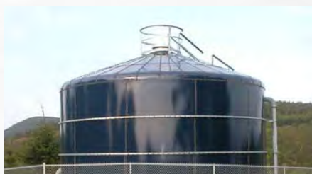
Knuckle Roof: Available on tanks up to model 31 diameter
