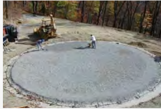
Ring Wall and Compaction
