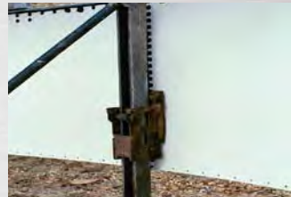
Set Up Jacks and Start Dome
