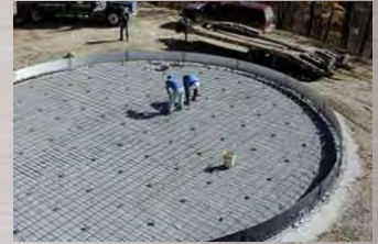
Set Slab Reinforcing Steel
