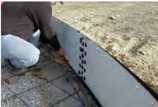
Install Water Seals
