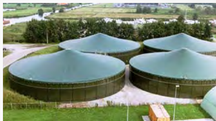
Fabric Roof: Economical, for low profile tanks in low wind areas
